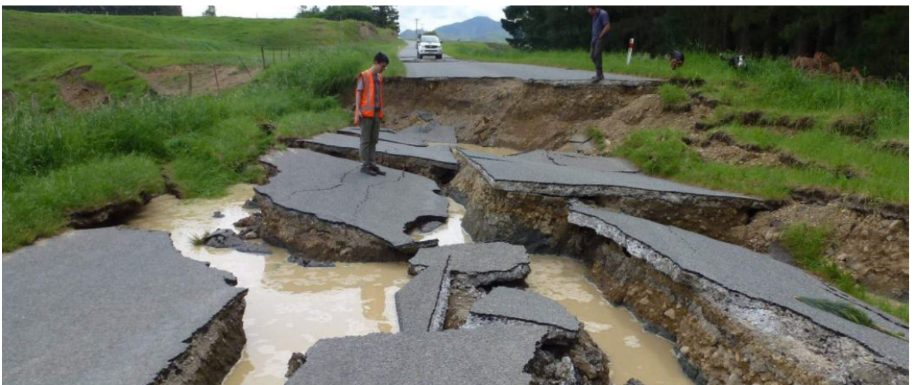
The fault rupture zone near Waiau, North Canterbury. Source: Tonkin + Taylor.
