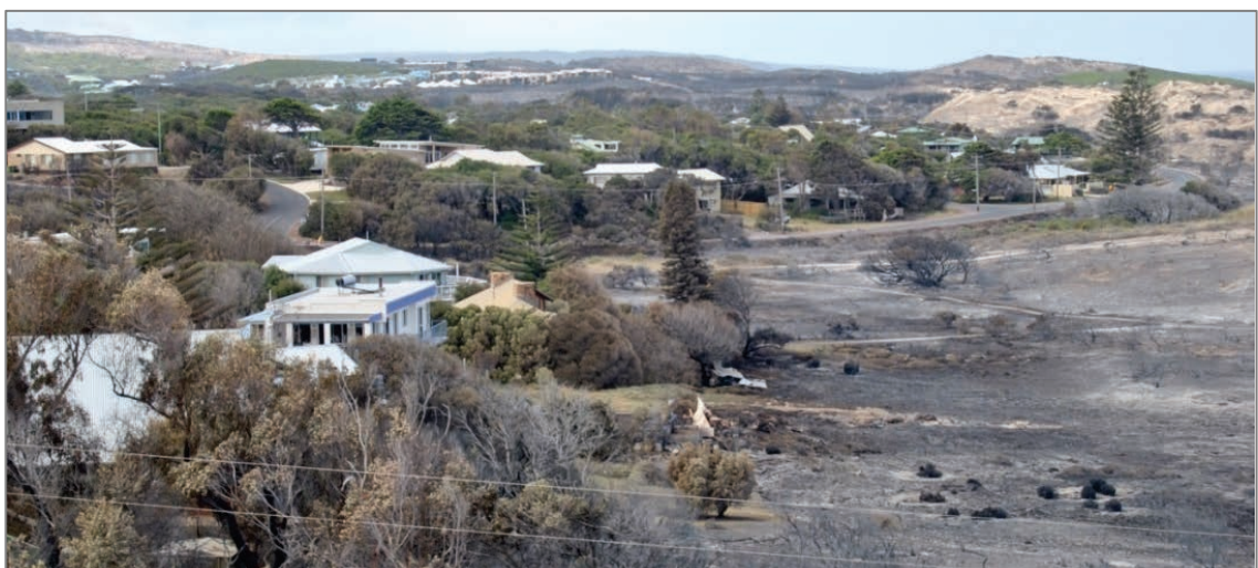
Figure 11: Structures damaged by fire (Source: Office of Bushfire Risk Management, WA)
