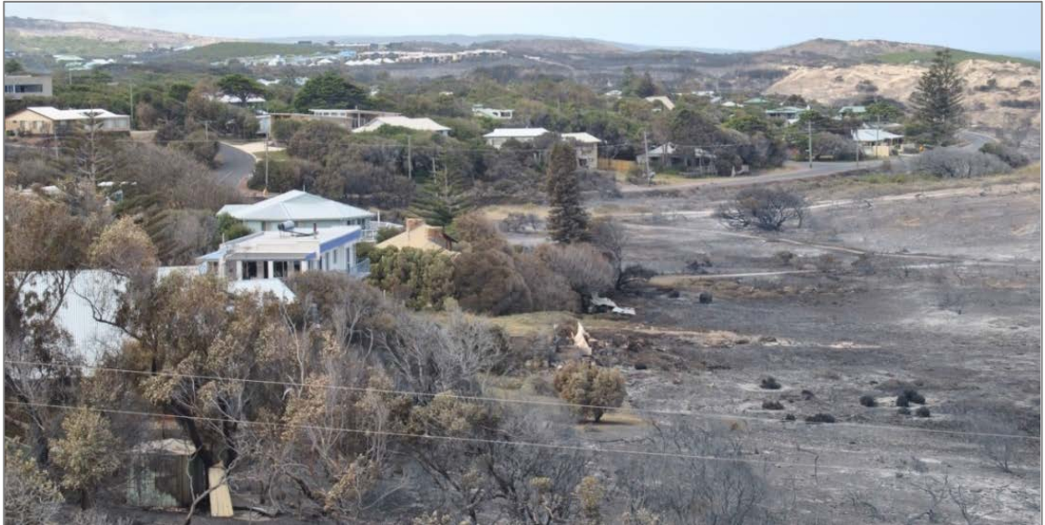
Figure 12: Structures damaged by fire (Source: Office of Bushfire Risk Management, WA)
