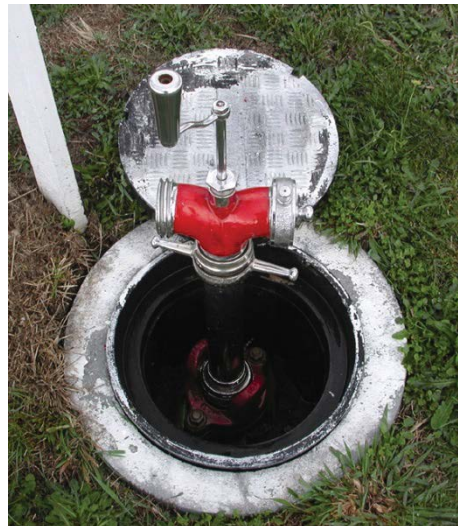
Figure 35: A typical below-ground hydrant with standpipe fitted
