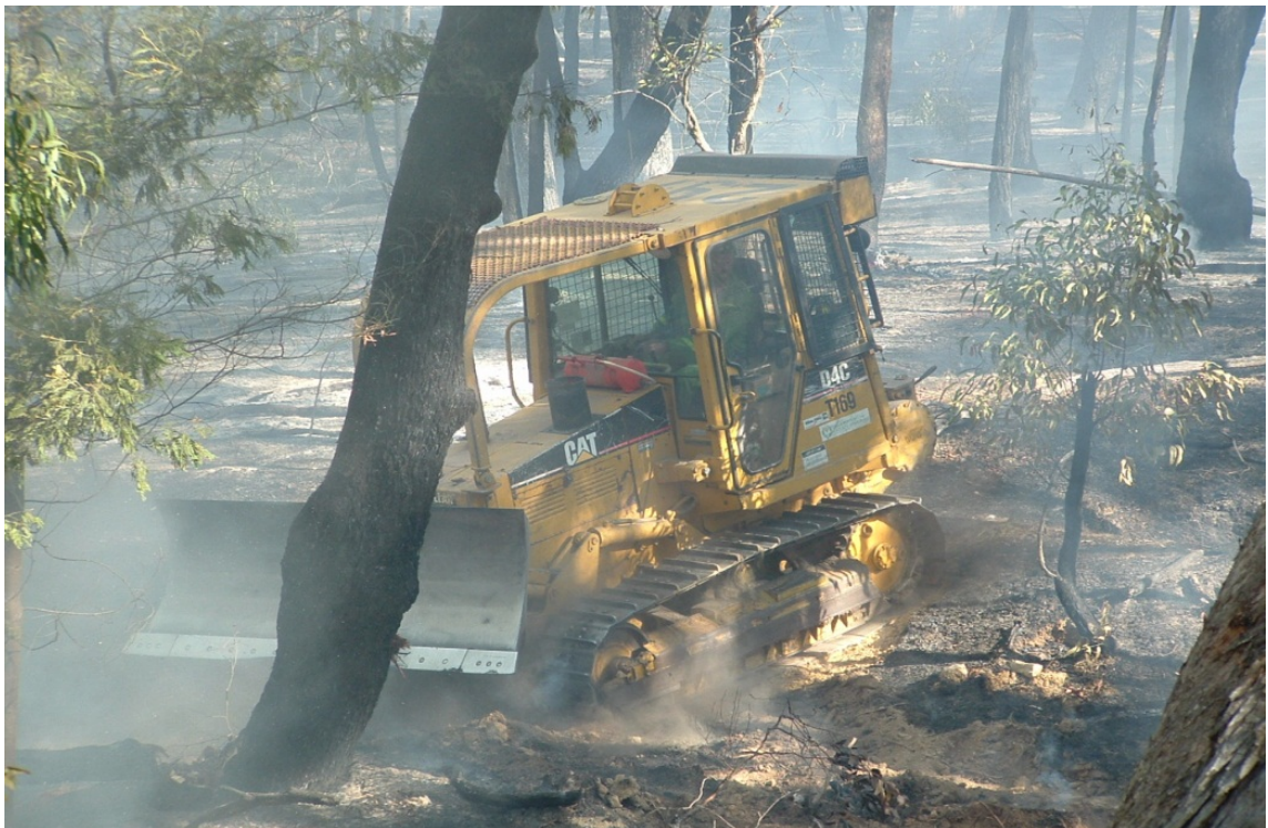
Figure 8: Bulldozer constructing fire-control line (Source: Bushfire CRC.)
