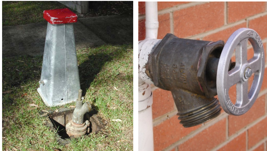
Figure 34: Types of above-ground hydrants
