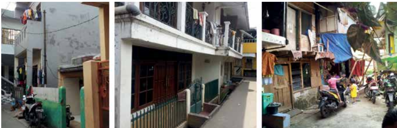
Figure 3: Two-storey houses with different quality of construction and materials.
