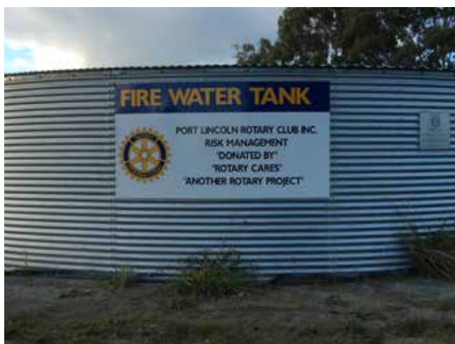
Community fire water tanks around Lake Eyre Peninsula are a constant reminder to people that the threat of fire is ever present.
