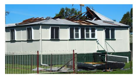
Figure 1: Severe structural roofing failure in Proserpine from Tropical Cyclone Debbie.
