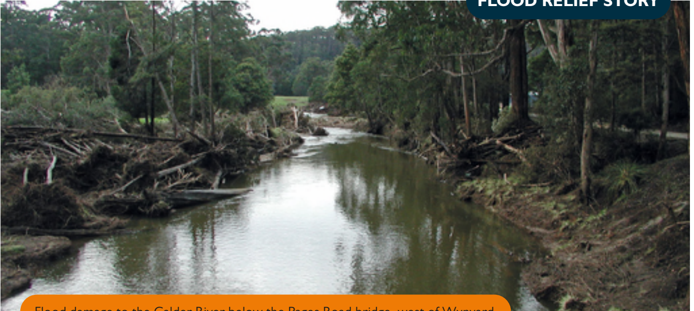
Flood damage to the Calder River below the Pages Road bridge, west of Wynyard
