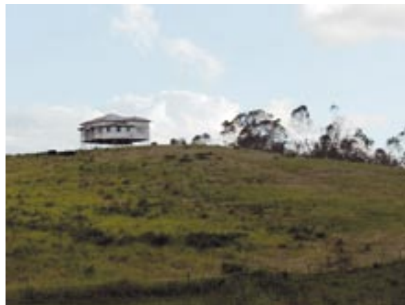
This isolated and seemingly vulnerable house, north of Innisfail, stood through the fury, although surrounding sugar cane was flattened; an example of the patchy wind speeds. Photo: Douglas Goudie
