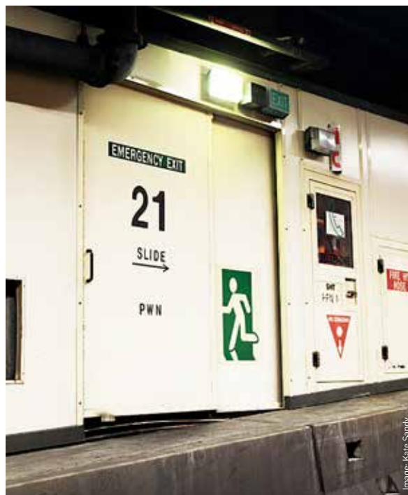
Impediments to evacuation. The jersey barriers had two small cut away steps (visible in bottom right of this photo) which the elderly participants were unable to use without assistance. They took around five seconds to climb the barriers with assistance.
