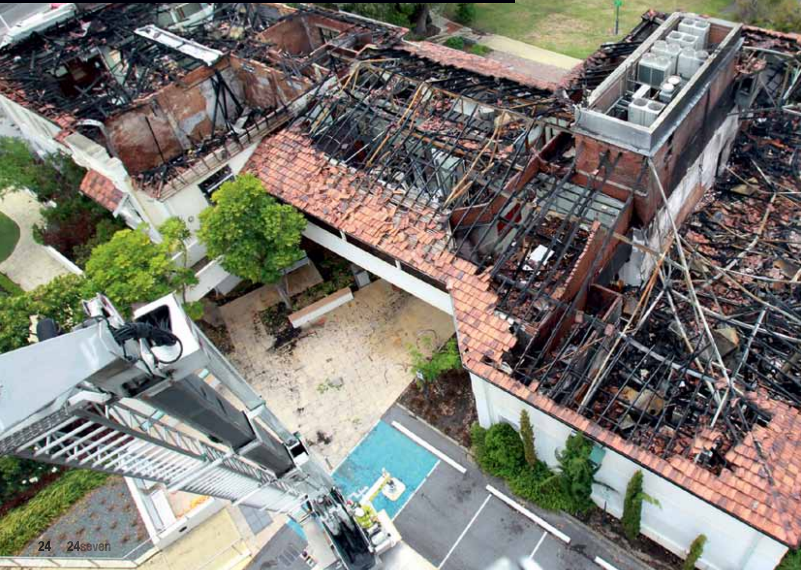
The collapse of the ceiling and intensity of the fire made it extremely difficult for crews to fight it from inside. Photo courtesy Perth Now .
