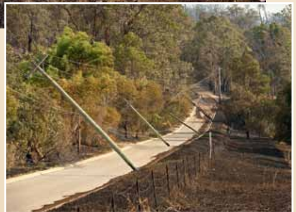
As the fire spread these power poles caught fire and fell onto the road.
