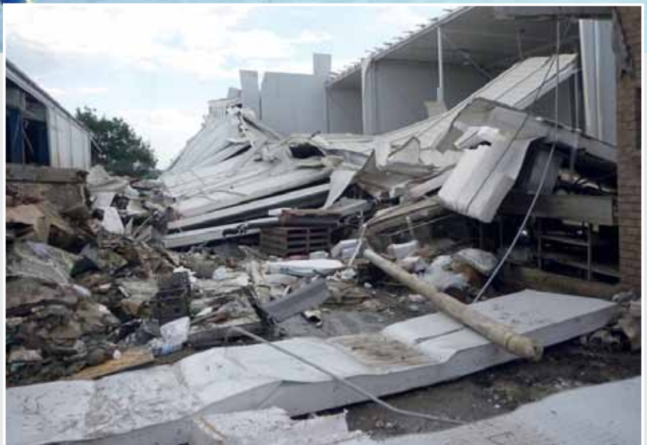
Top: Members of the national USAR Taskforce prepare for deployment in Queensland. Above: Some of the extensive damage caused by floods in the industrial area of Rockley.
