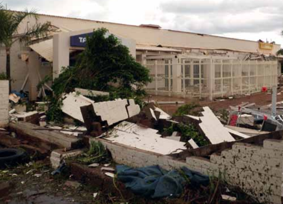
Tornado damage at Karratha's Mercure All Seasons Hotel.
