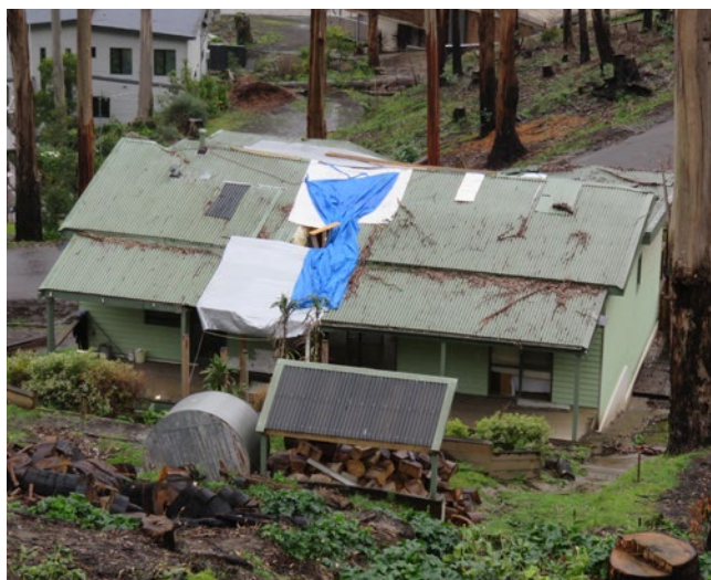
Figure 3: A house on Wallace Street, Wye River damaged by tree strike caused by fire.
