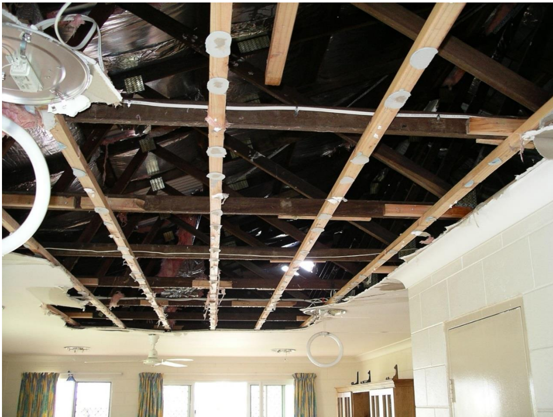
Figure 28. Damage to ceiling and fittings from wind driven rain via in part debris damage to gable end (TC Larry)
