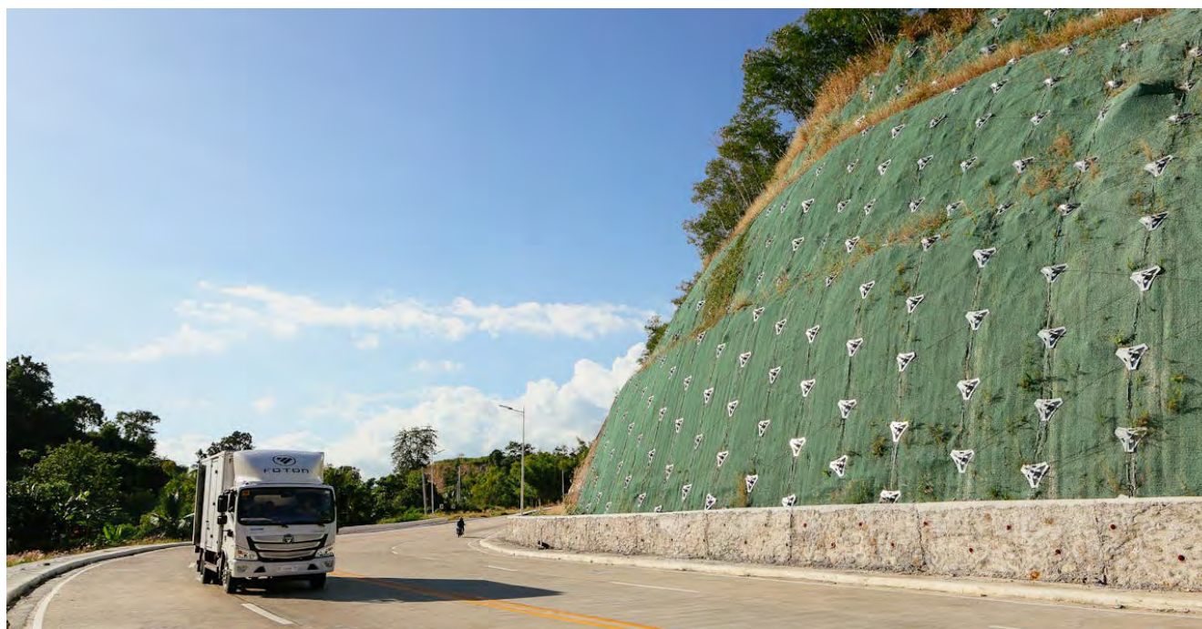
Figure 3: Vegetative filter strips/turfs for flood and erosion mitigation.
