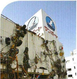
Fishing nets wrapped around buildings in Shizugawa by tsunami
