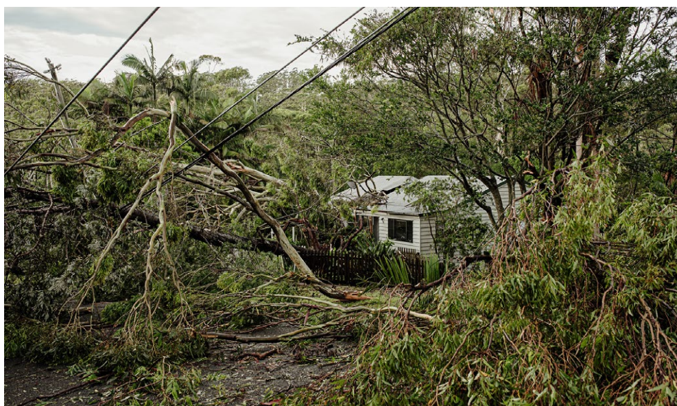
A tornado caused significant damage to houses, roads and power infrastructure in the Tamborine Mountains, Queensland in 2023.
