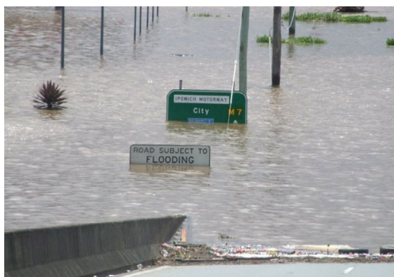
Major Brisbane highways were cut by flood waters in 2011.
