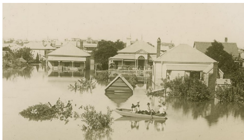
Submerged houses in South Brisbane after 1893 flood. Source: University of Queensland.
