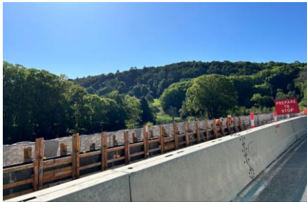
Road repairs, Northern Rivers, after 2022 floods. Taken 2/9/2024
