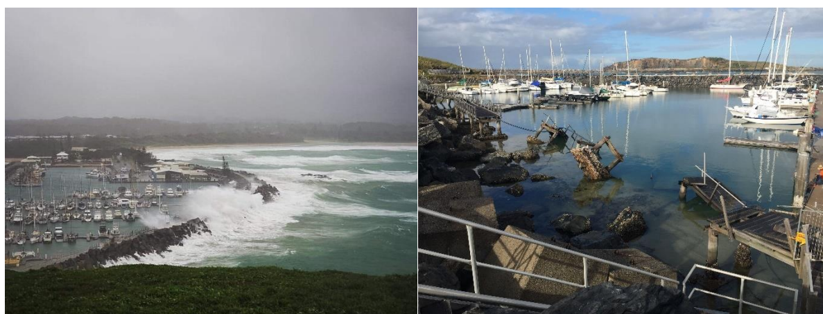
Figure 3: Breakwater at Coffs Harbour during storm and damage to marina walkway.
