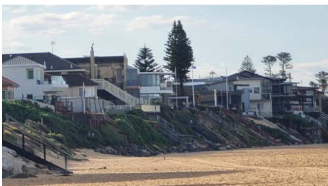
Legacy development on the eroded beachfront of Wamberal, New South Wales.
